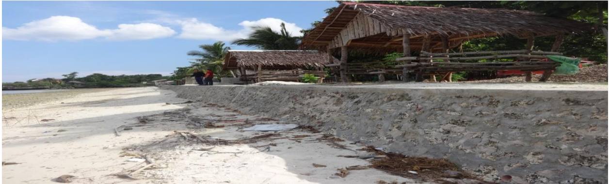
CAMOGAO : Construction of Camogao Seawall ( Fully Functional )
