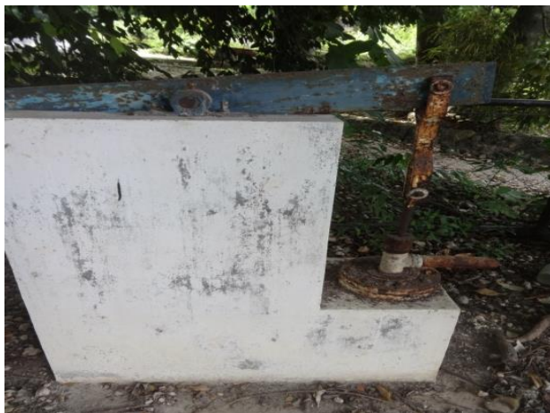
POBLACION : Installation of Poblacion Level I Waterworks System ( Totally Not Functional )
