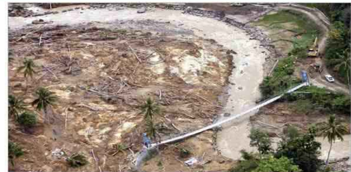
In an affected area where all houses and infrastructure were destroyed because of the earthquake that hit Padang on September 30, 2010, bridge built under PNPM-Rural survived the disaster.
