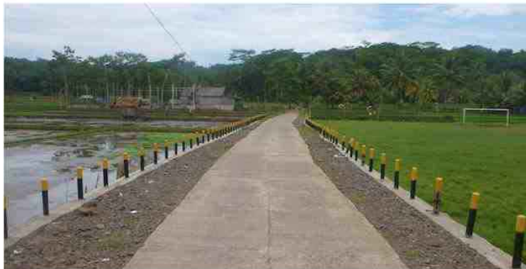
Concrete Road in Aceh
