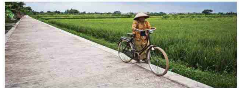
Concrete roads such as this one in Java built under Rekompak increased mobility of villagers and improved quality of life by providing easier access to markets, schools, farmers' fields, and homes of friends and relatives. They also provided faster escape routes in case of disaster.
