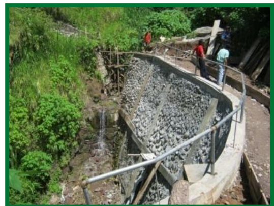
Figure 4 - Example of a slope protection subproject in KC taken (Iloilo)
