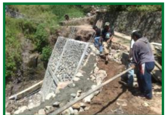
Figure 12 - Example of slope protection using riprap methodology
