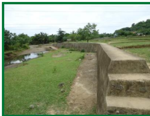
Figure 22 - Example of the Camarines Sur river protective structure that was developed to stop seasonal flooding resulting from the overflow of the river
