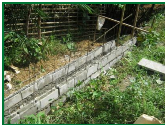
Figure 8 – An example of a lateral improvement that transports localized flooding in the municipality
