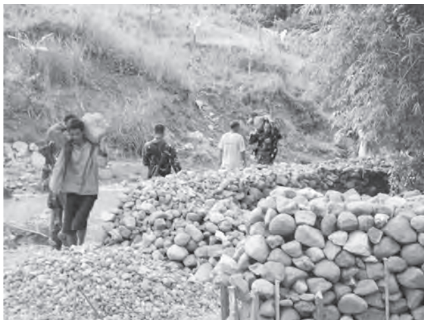
SOLDIERS and villagers pile the stones near the construction site
