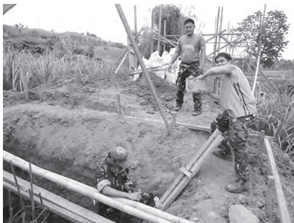
SOLDIERS dig holes for the bridge’s posts
