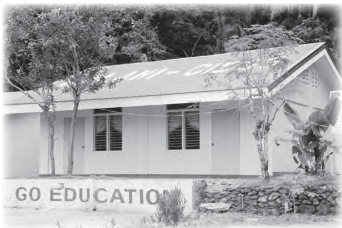
The school building constructed by Kalahi-CIDSS in Barangay Talisay in Calatrava, Romblon
