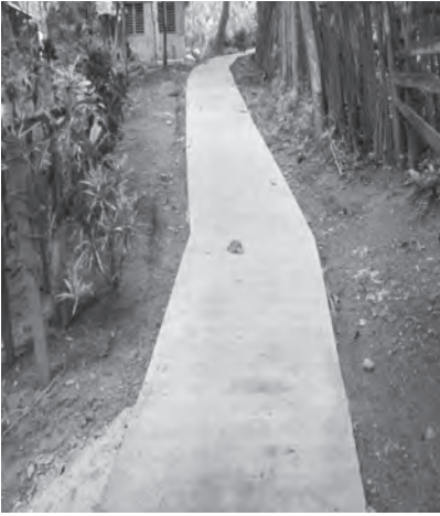
The pathway to peace in Barangay Sulo in Naga, Zamboanga Sibugay, constructed through Kalahi-CIDSS PAMANA
