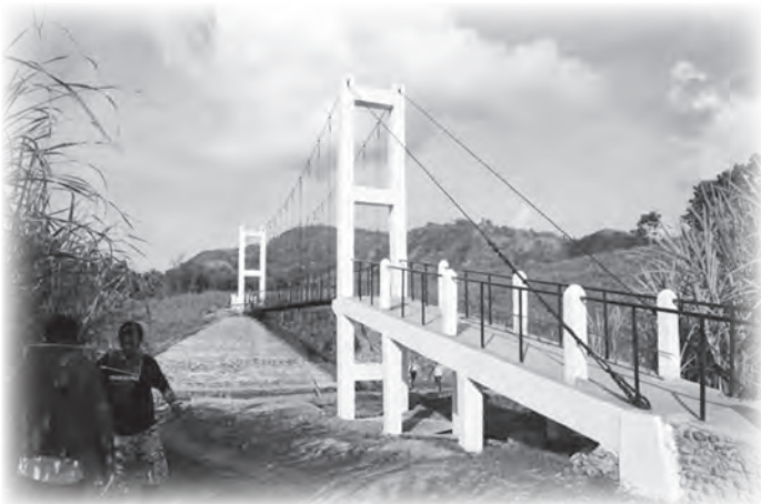
BRIDGE OF UNITY – the Bandila hanging bridge symbolizes the trials and triumph for community volunteers in realizing the project
